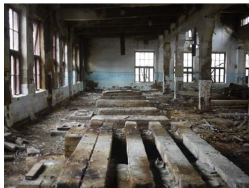
TNT washing building after equipment removal (Source: Pure Earth)
